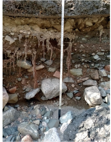
Figure 7. The formation of erosion of the slopes of the roadbed on area 4
