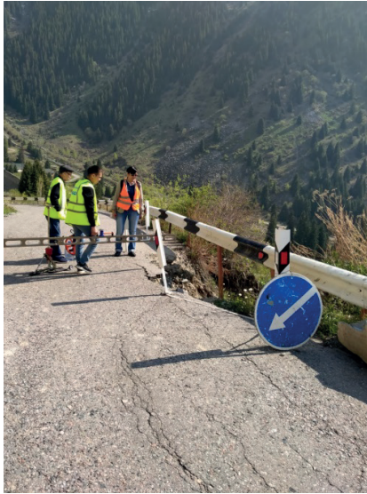
Figure 7. The formation of erosion of the slopes of the roadbed on area 4
