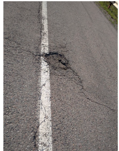
Figure 8. Small cracks and pits that appeared on the surface of area 5
