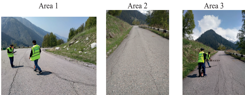
Figure 6. Longitudinal and transverse cracks formed on the surface of the automotive coating in areas 1-3
