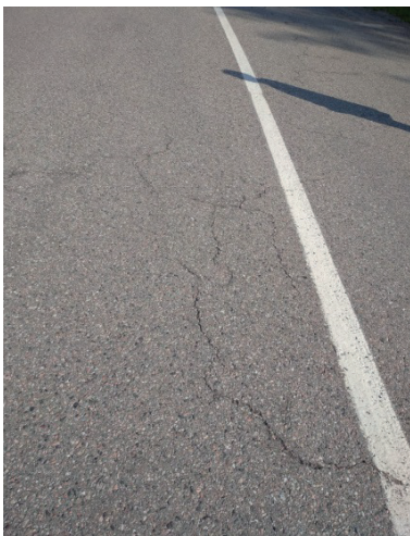
Figure 8. Small cracks and pits that appeared on the surface of area 5
